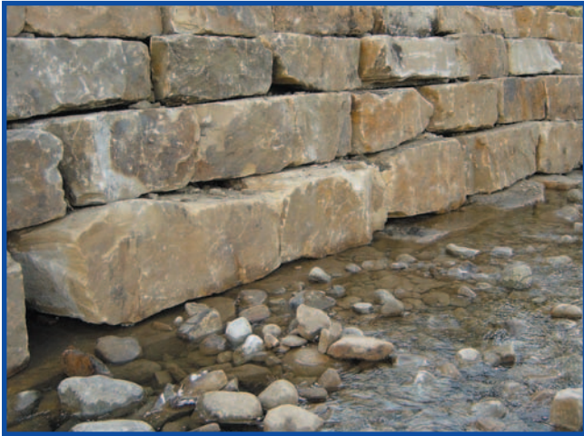
Above: When submerged, stone revetting provides stable refuges for crayfish.
