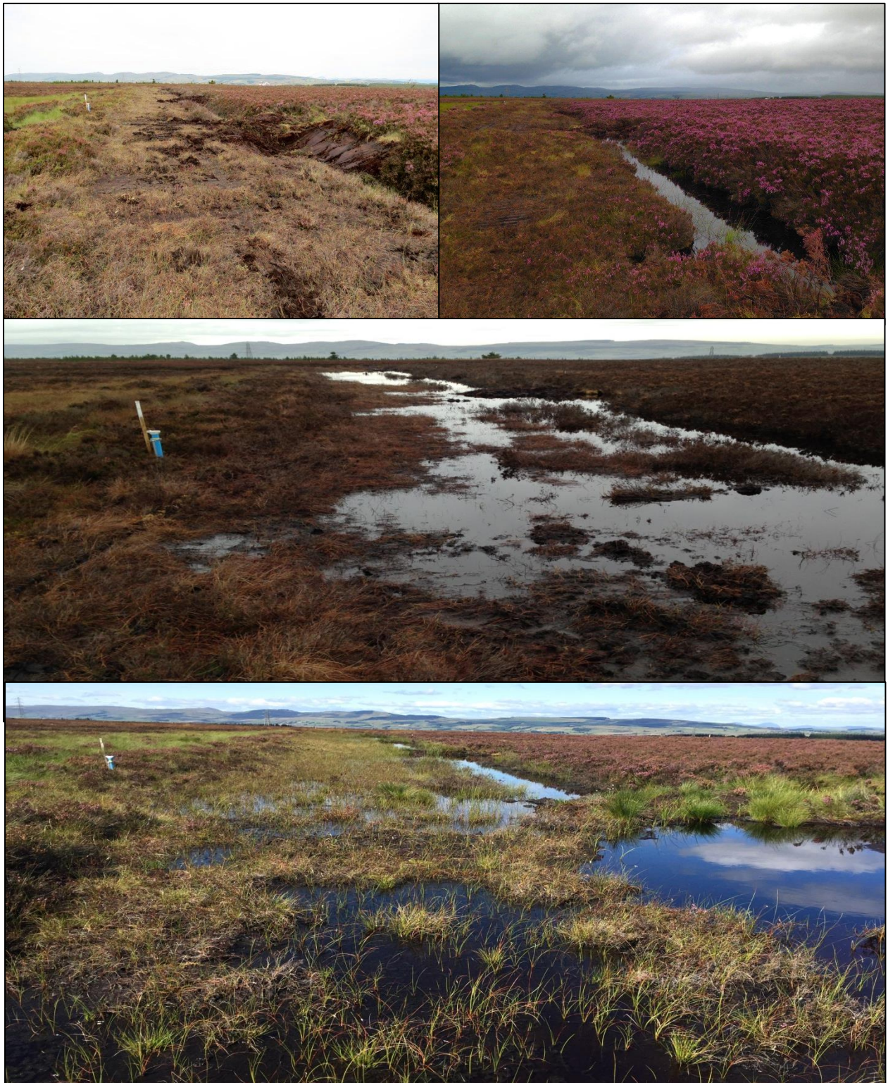
Figure 2. Peat dams on ditch between Compartments 7 and 8.
