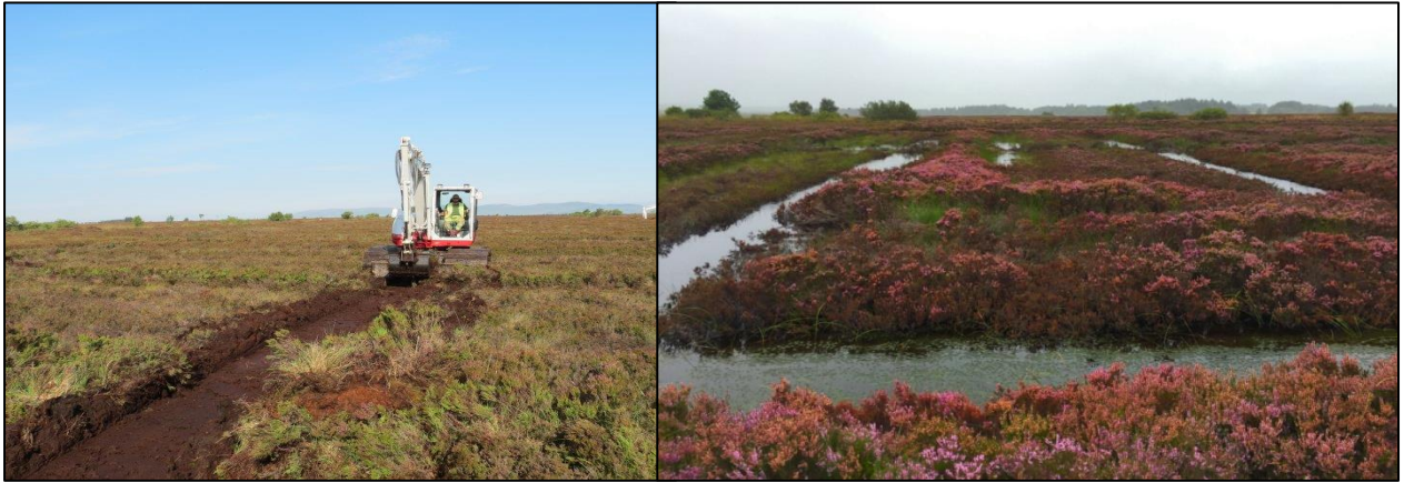
Figure 1. Installation of linear trench bund in Compartment 13a.
