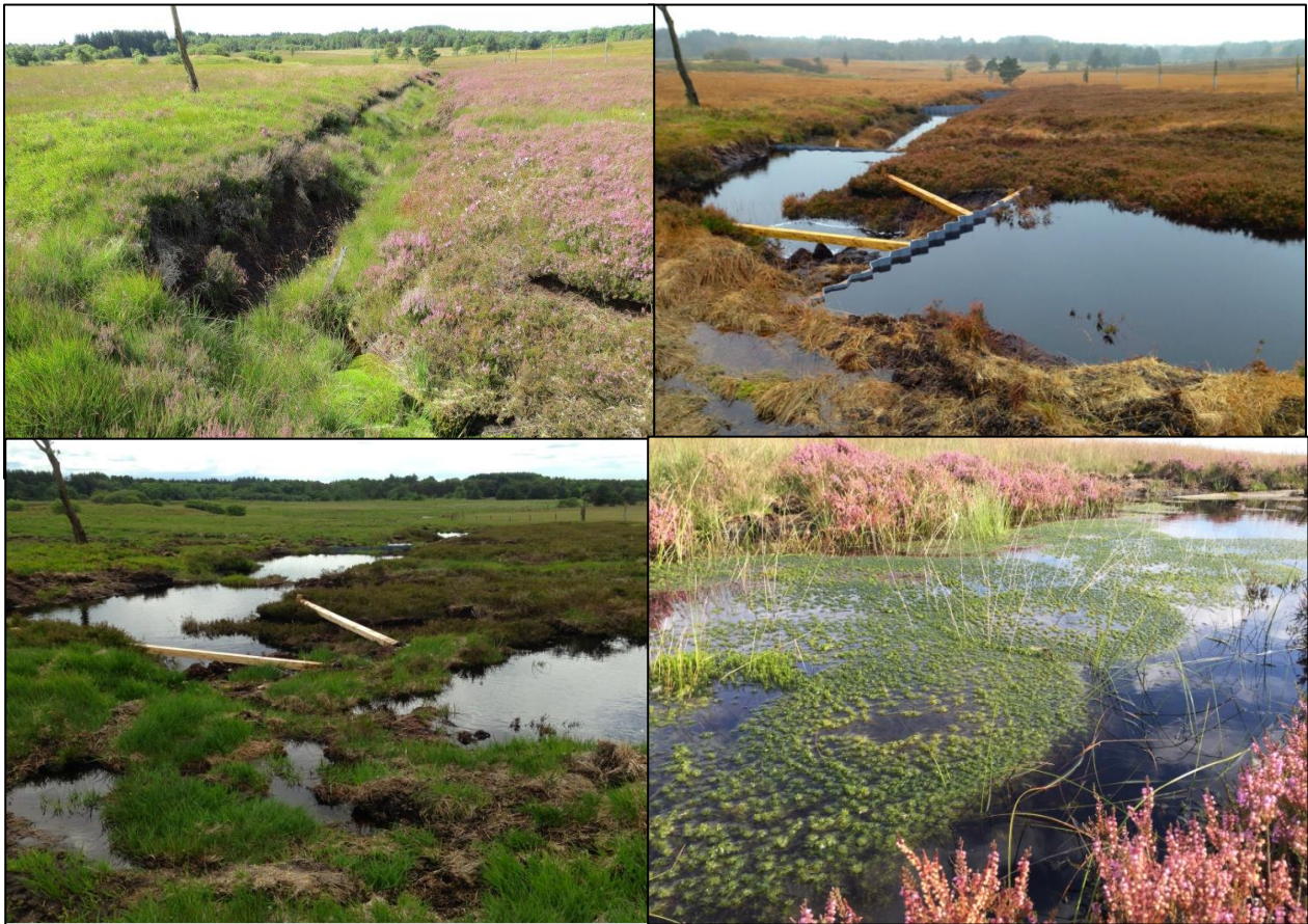
Figure 4. Large ditch in Compartment 2 at Fannyside Muir before and after installation of reinforced plastic piling dams.
