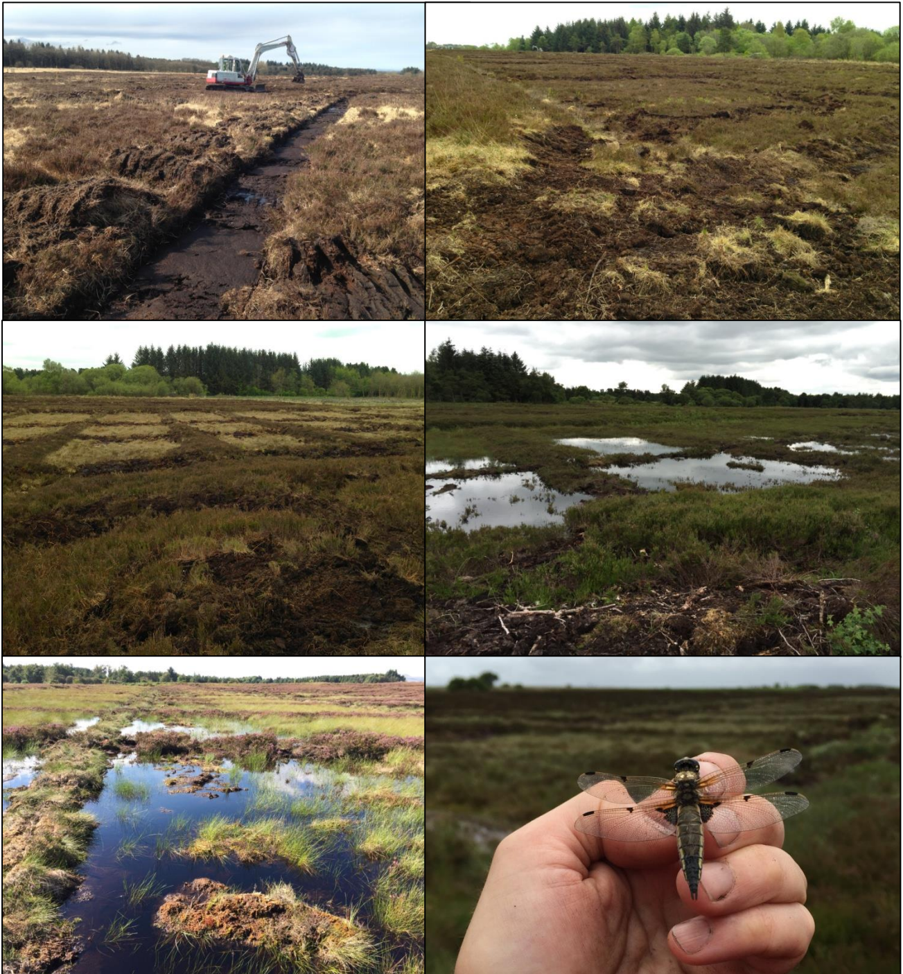
Figure 3. Installation of cell-bunding in hand-cut area of Compartment 1
