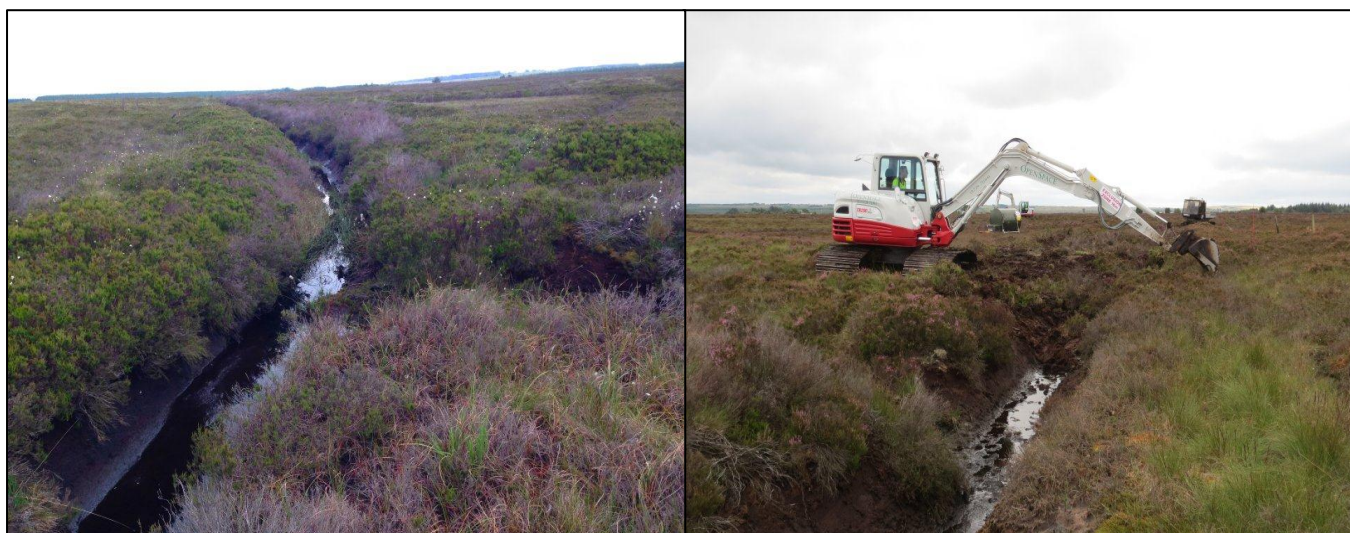
Figure 5. Reprofiling steep-sided boundary ditch.
