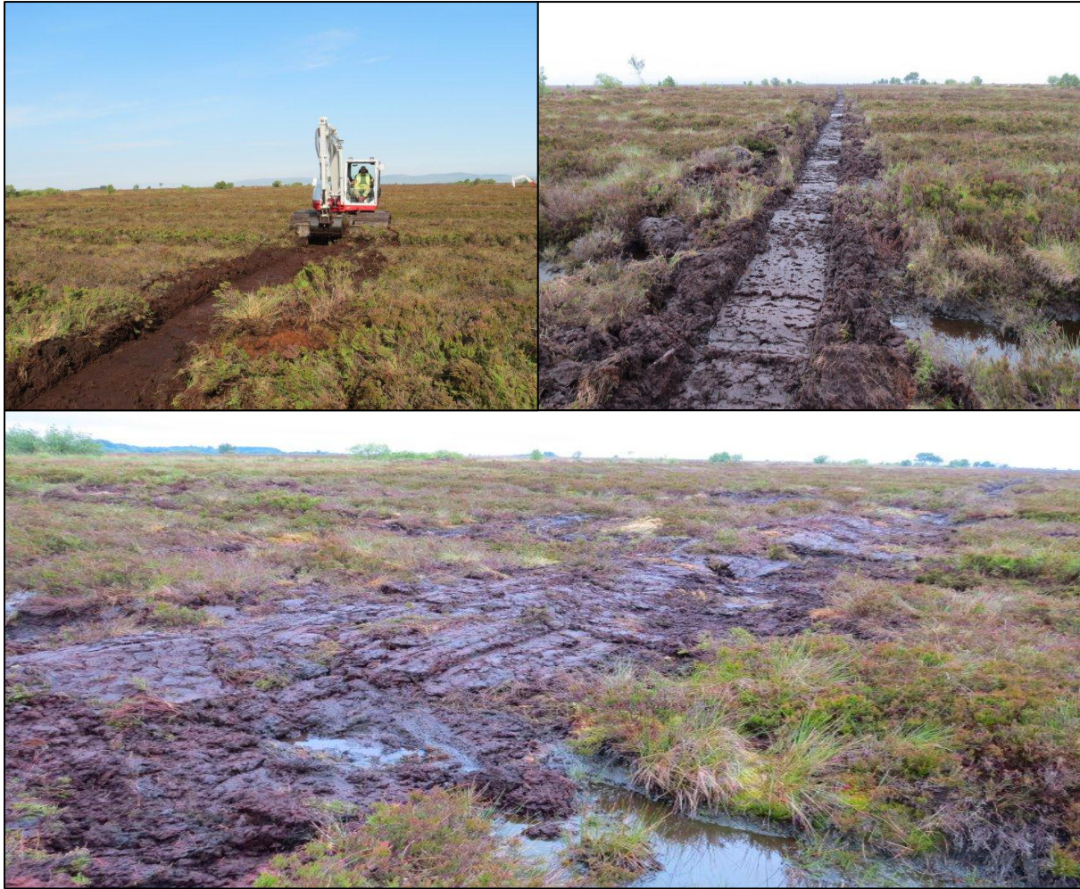
Figure 1. Installation of trench bund in Compartment 13a.
