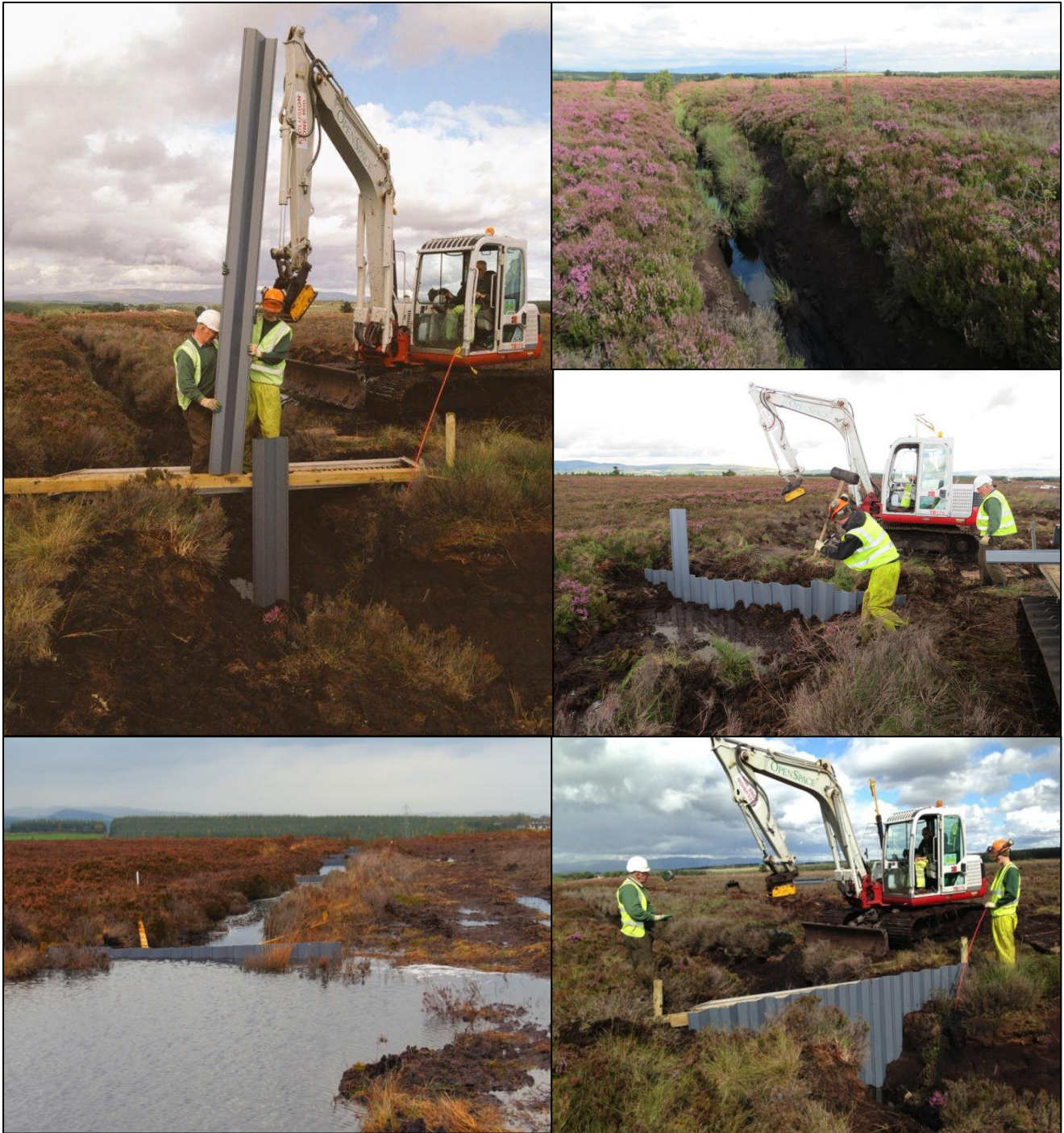
Figure 3. Installation of 4m deep plastic piling dams on large ditch between Compartments 5 and 6 at Fannyside Muir.
