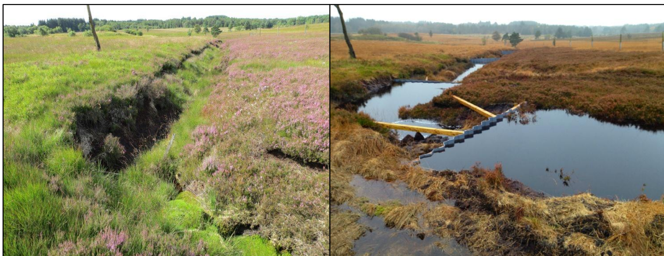
Figure 4. Large ditch in Compartment 2 at Fannyside Muir before and after installation of reinforced plastic piling dams.
