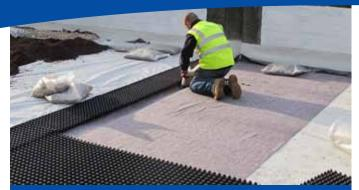
Above: Biodiverse roof installation showing the root barrier, drainage board and filter fabric
